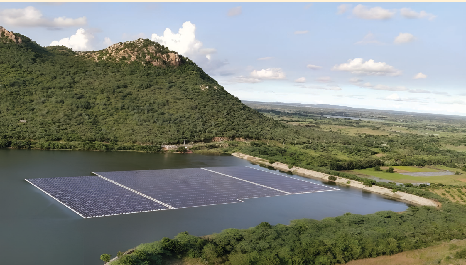
Image 19: A 4-megawatt floating solar plant commissioned as part of SCM in Tirupati (Andhra Pradesh). Source: Tirupati Smart City
