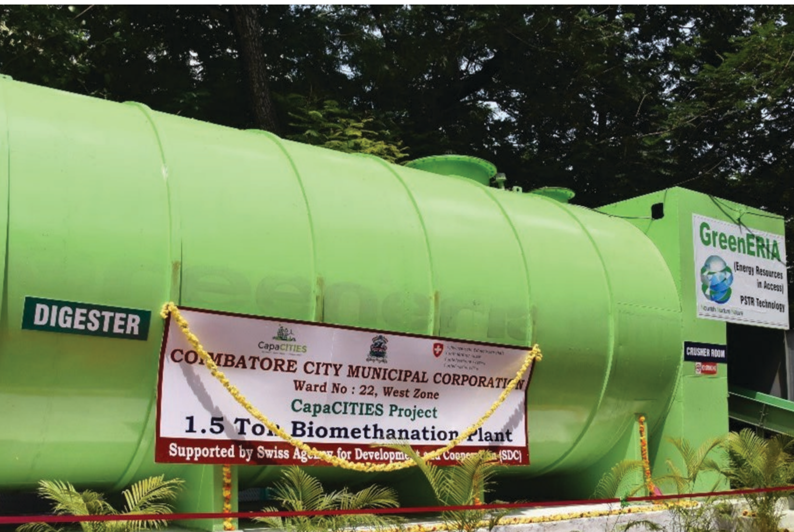
Image 21: The bio-methanation plant commissioned by Coimbatore Smart City produces approximately 60,000 m 3 of biogas and 39,055 m 3 of methane annually, generating around 7 KW of electricity per day. Source: Coimbatore Smart City.
