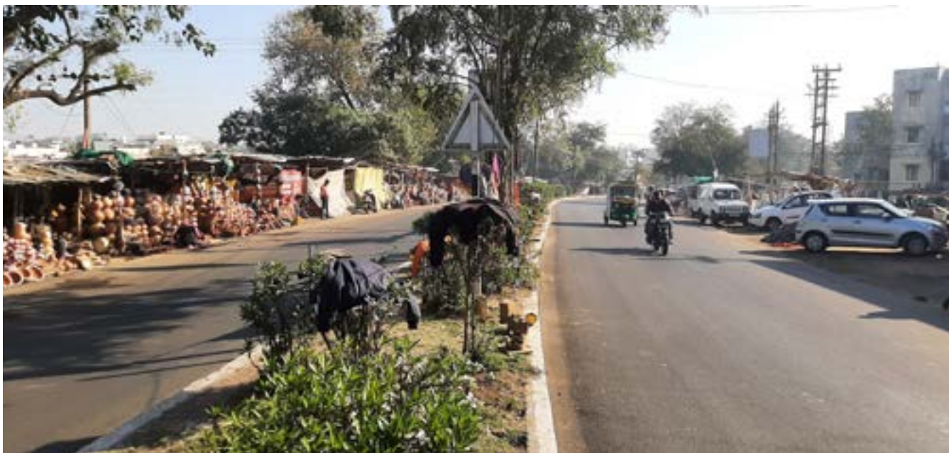
IMAGE 3.12 Encroachment along MANIT Chouraha, which has no footpaths or cycling lanes
