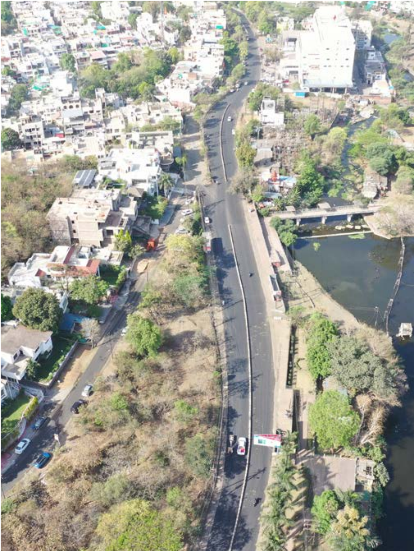
Chunabhathi Road with Shahpura lakefront on the right and Pahadi Mandir forest patch on the left.
