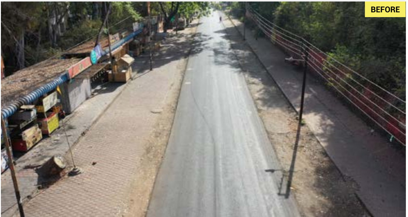
FIGURE 3.23 Before and after illustrations of pedestrian street development along Campion School Road
