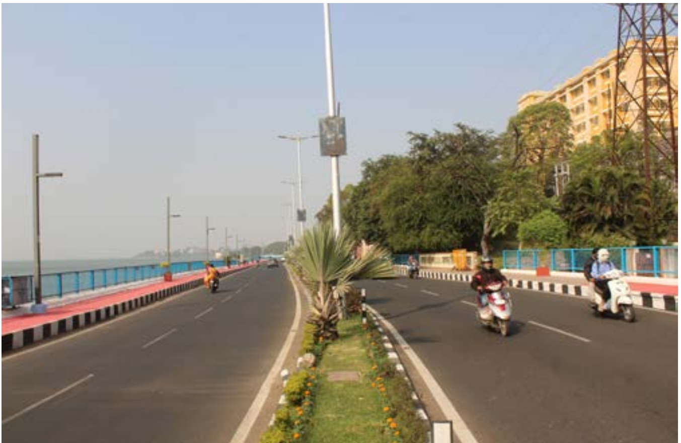
IMAGE 3.4 VIP Road along the northern banks of Upper Lake
