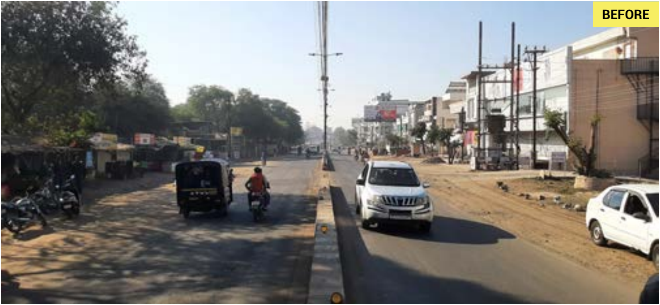
FIGURE 3.22 Illustration of application of Complete Streets Framework along Kolar Road to develop it as Eco-arterial Street.
