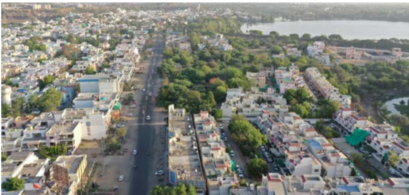
IMAGE 3.13 Lack of footpaths or cycling lanes along Kolar Road
